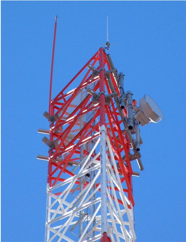
**Fig. 5.** 7 GHz microwave dish on 50 meter Malargüe comms tower.
