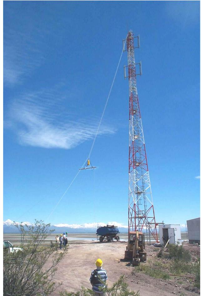
**Fig. 4.** Panel antennas on 41 meter Los Leones comms tower.
